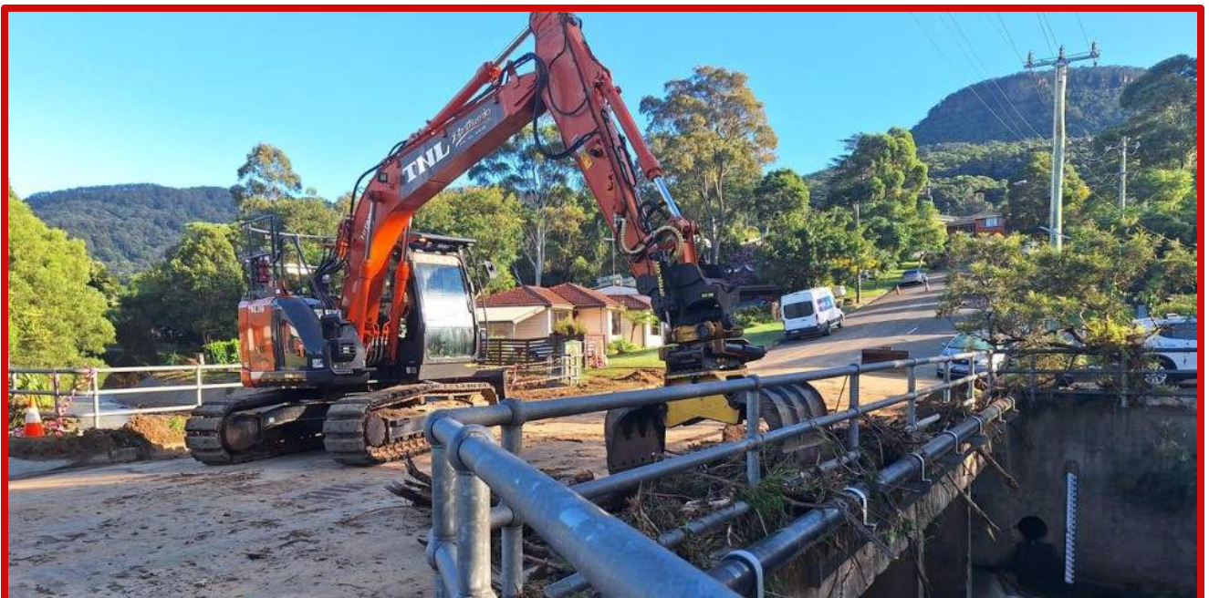
Cleanup works on Koloona Avenue, Figtree, April 2024.
